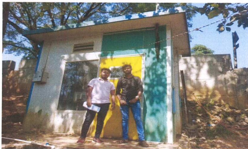
Fig: Inspection of R.O Plant, Adyaru
