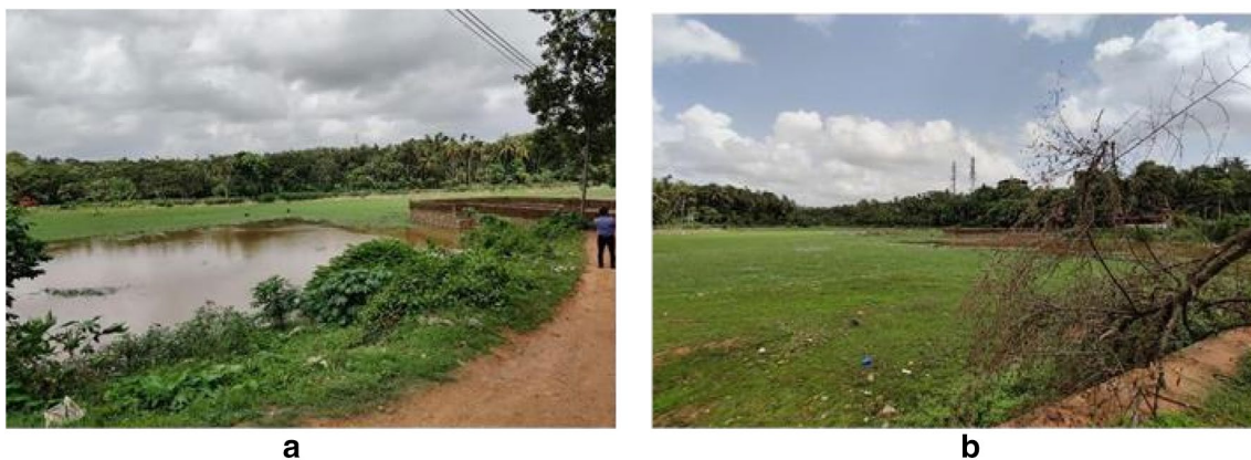
Fig. 2 Existing condition of the lake a east side b west side
