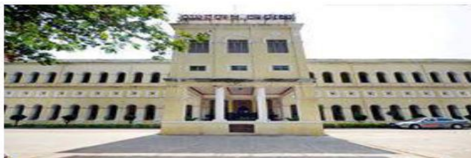
Fig 5: Front view of Yuvaraja College of Mysore for which Seismic evaluation is performed
