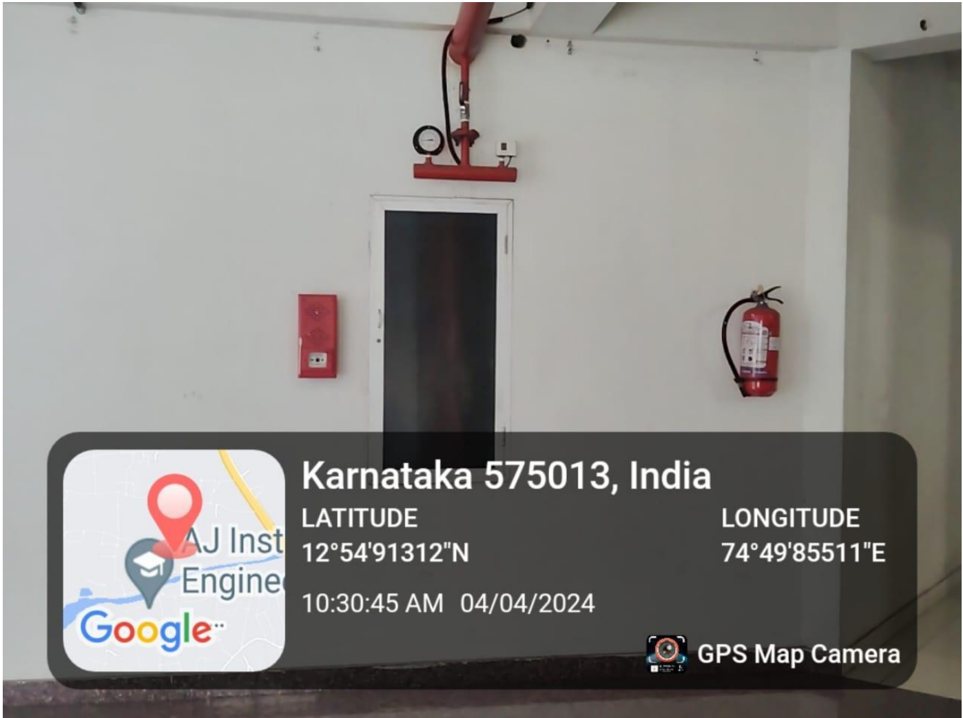
Fire Safety in Girls Hostel
