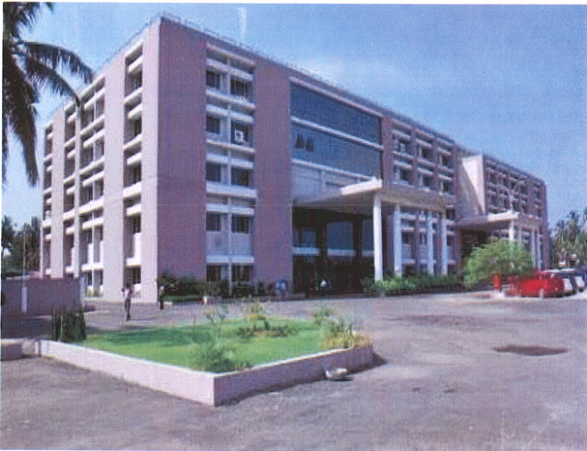
Fig 1: Front view of A J Institute of Engineering & Technology
