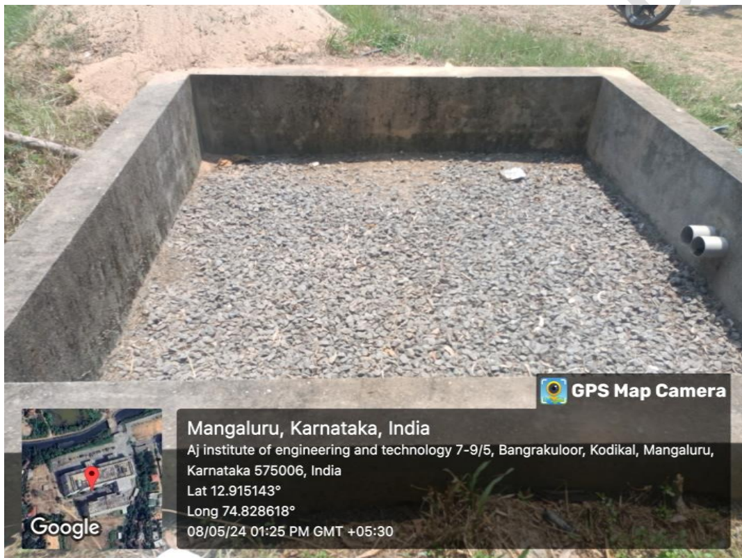
Plate 6: Under process rain water bunds in the premises
