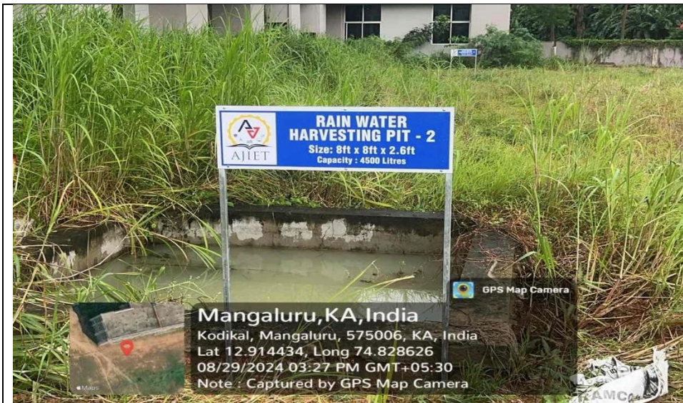
Rain Water Harvesting Pits
