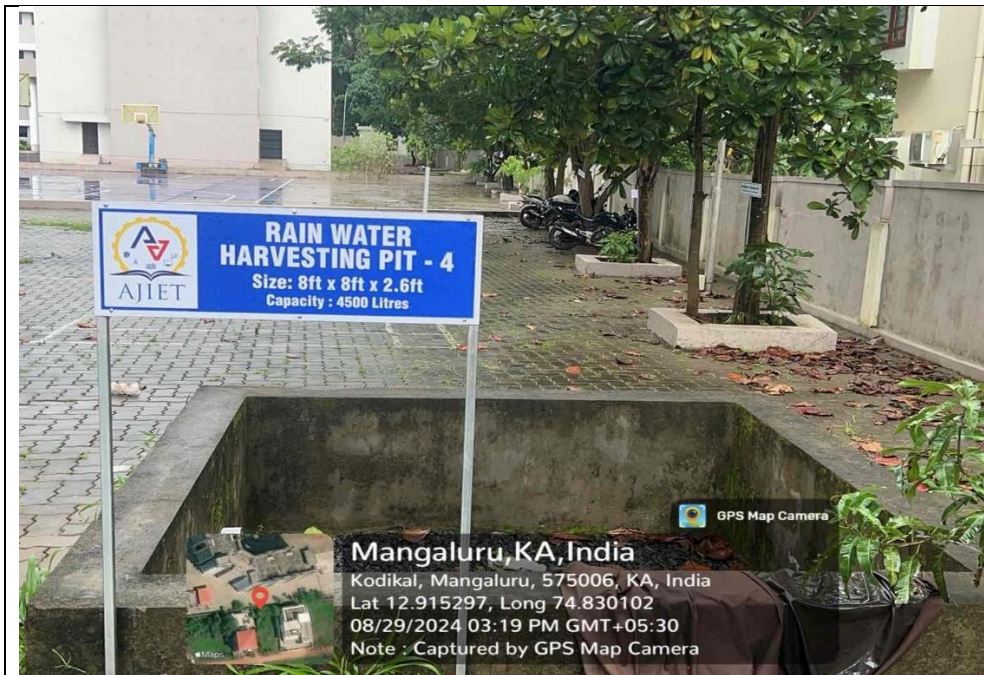
Rain Water Harvesting Pits
