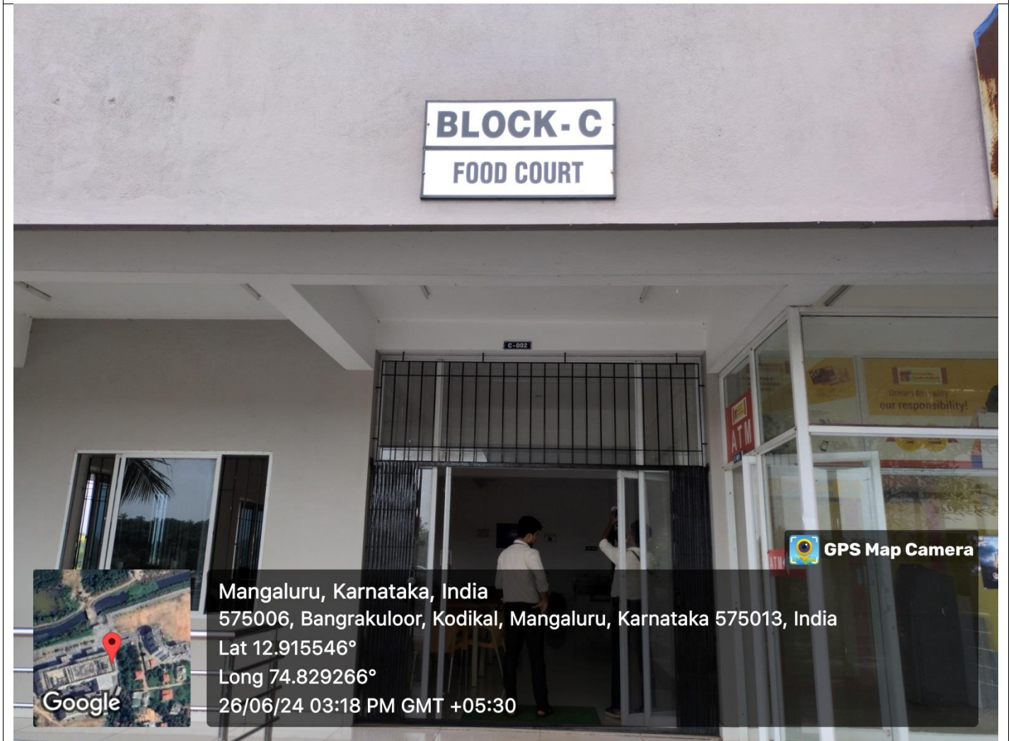
CAFETERIA-2 FRONT VIEW
