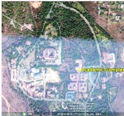
Fig. 7.6: Satellite imagery of Indira Gandhi National Open University campus at New Delhi. Place mark shows the New Academic Complex (source: www.earth.google.com)
